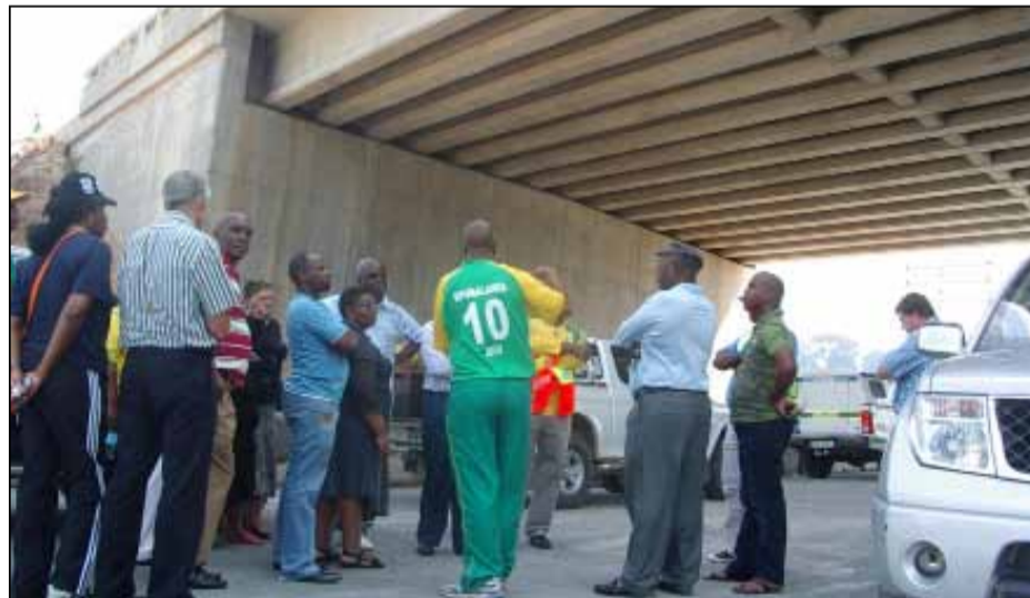
A parliamentary delegation inspect the bridge near Nelspruit that collapsed on September 30 last year. In the green shirt and pants is Mathew Mohlasedi, head of the Mpumalanga department of public works, road and transport
