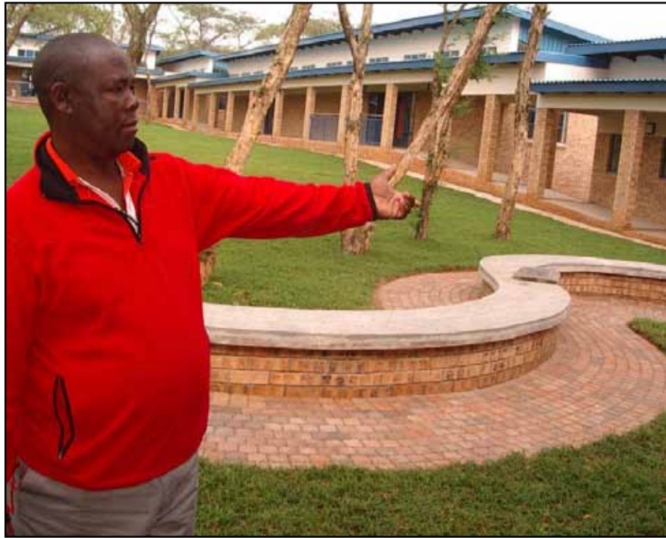
READY BUT EMPTY: The site agent for Clear Choice Builders, Andries Mkhethwa, on the grounds of the completed John Mdluli Primary School. Pupils cannot move in because there is no water yet
