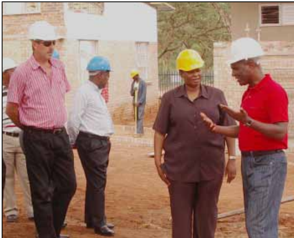
Spokesperson for Clear Choice Builders, Joe Manonga talks to Mpumalanga education MEC Rejinah Mhaule on Monday about the rebuilding of two schools that were demolished to make way for a parking lot at the 2010 soccer stadium in Nelspruit.
